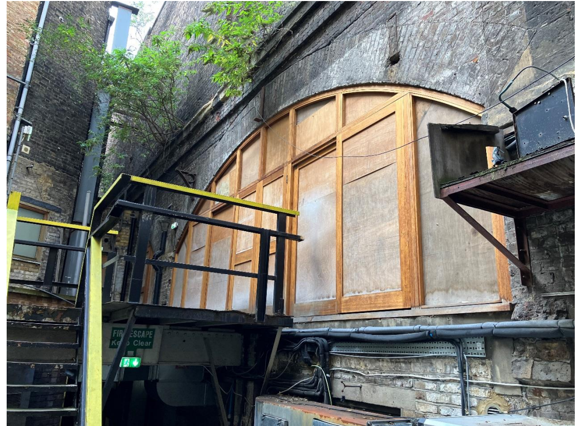
Existing rear archway and escape stairs
